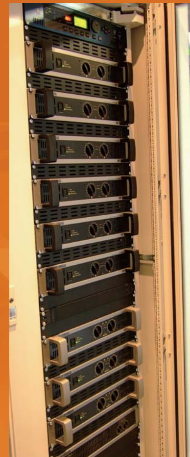
The well-equipped rack with the Yamaha DME24N and the Yamaha amps
