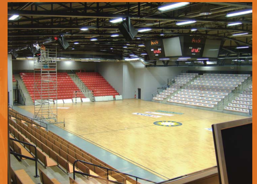
Inside the arena showing the score boards and the suspended Yamaha IF2115 installation directed towards the stands.
