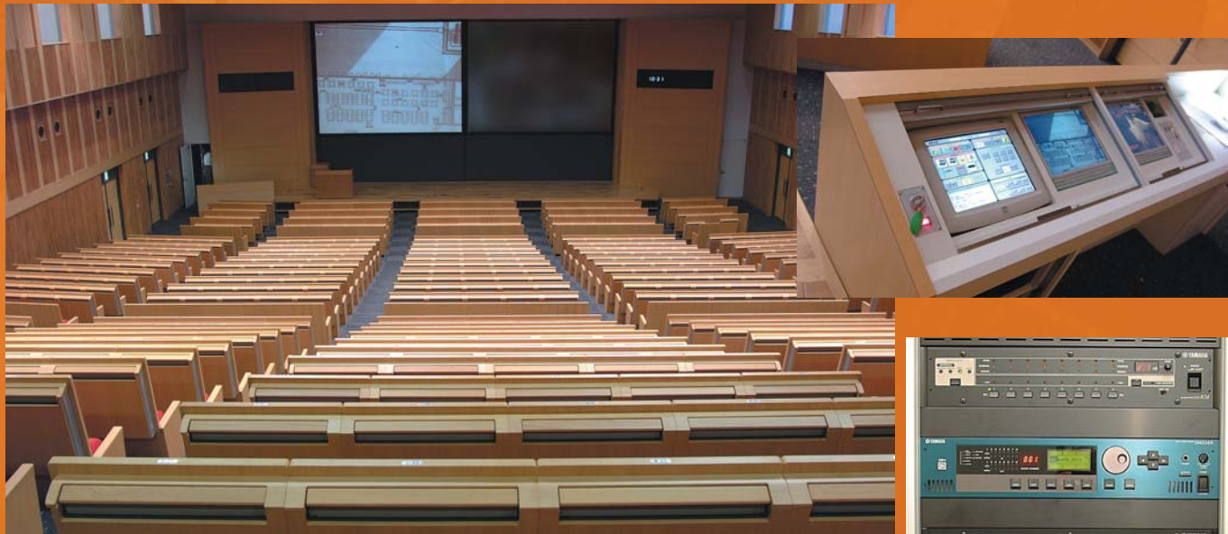
This lecture hall on the 1st floor of the new structure is the largest, providing seating for up to 600 students. It features a DLP projector and 300-inch screen, plus an additional two LCD projectors and 250-inch screens. Easy operation is provided via touch-panel controllers.
